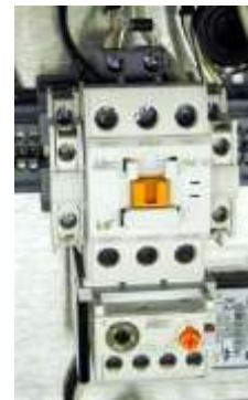
Figure 12. Motor Contactor
